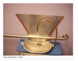
A toilet modification that allows users to save water by utilizing the wastewater from handwashing to flush the toilet.
